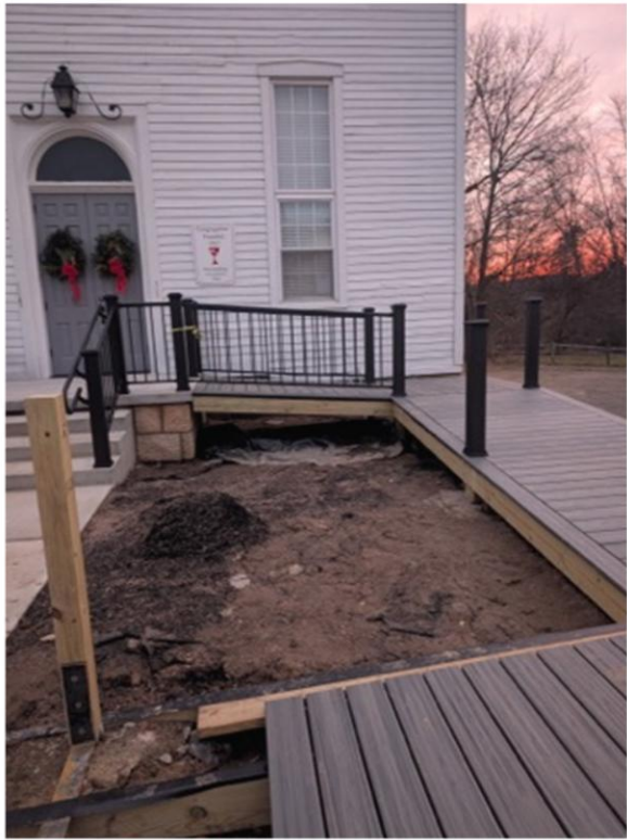
The ADA compliant ramp begins to take place!
