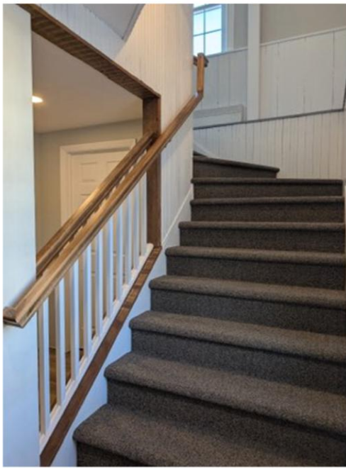
Carpeting on our finished steps!
